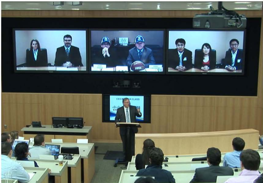
The virtual lecture hall at the Fuqua School of Business at Duke University features a custom-built integration of Cisco TelePresence. Its features include three 103-inch plasma displays, six 1080p cameras, an instructor's podium with two document cameras for content, three remote student displays for the instructor to view remote classrooms from the podium, and 66 custom push-to-talk microphones for interactive discussions. The system was built by systems integration partner IVCi.
